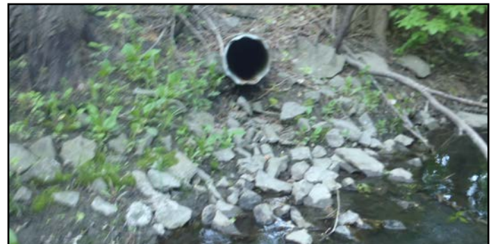
Section of Hunt Club Creek where unmitigated stormwater input elevates conductivity levels near Uplands Drive (above) and the stormwater pond outlets onto the creek upstream of Riverside Drive (below) lowering conductivity levels
