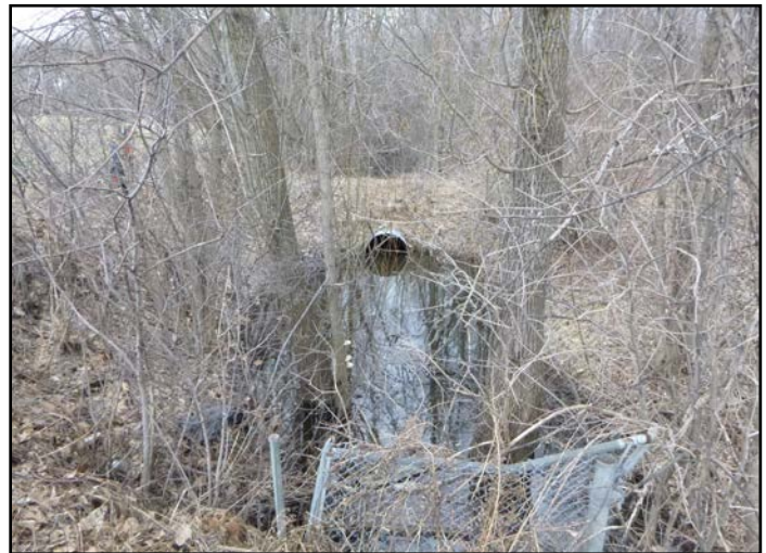
Piped headwater drainage feature on Hunt Club Creek, shows the upstream portion (above) buried and the downstream outlet remains open (below)
