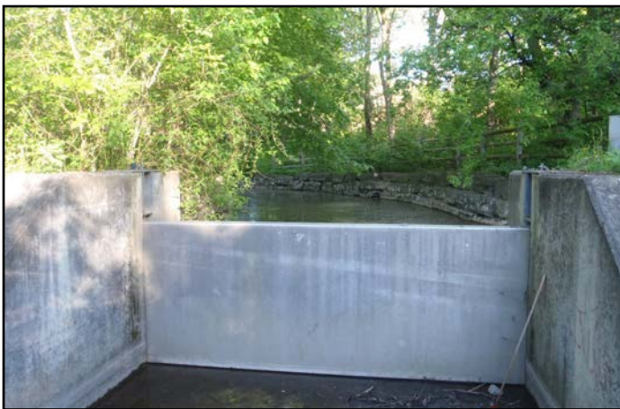
This water control dam on Hunt Club Creek creates a permanent migration barrier to fish communities
