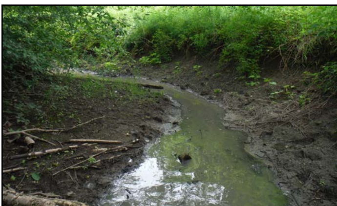
Bank erosion along Hunt Club Creek east of Riverside Drive
