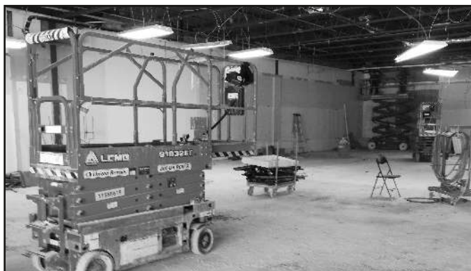
June 22: Gutting of inside
